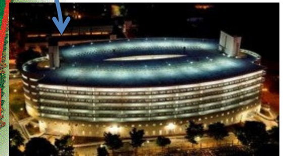
Multi Level Car Park 1100 cars
