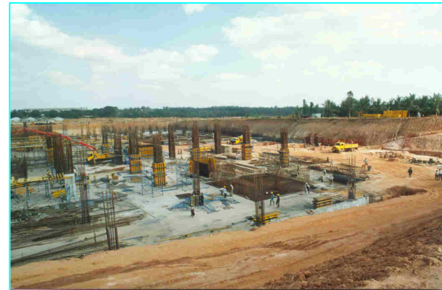
Construction site of ITPB October 1995
