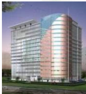
Multi-tenanted Building (Under construction)
